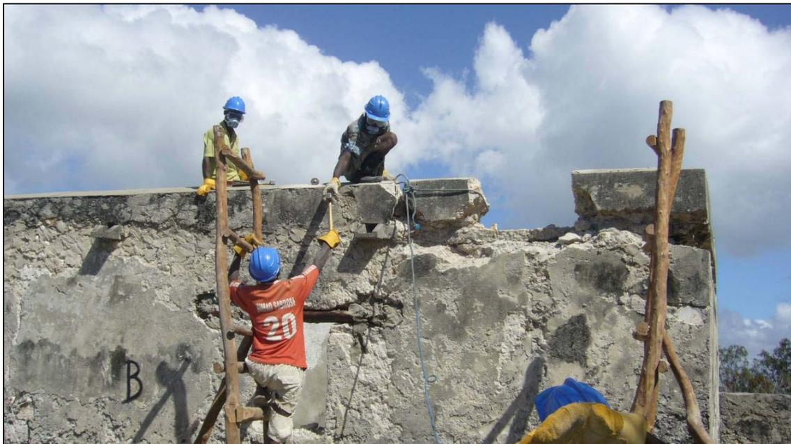
*From top left:* Securing rooms in the fort; painstaking removal of inappropriate iron reinforcements from the structure; dismantling fragile members before stabilizing the structure.
