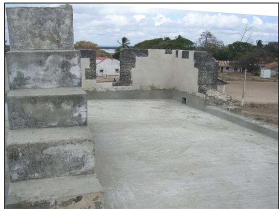
**Top row:** Collapsed battery and roof slab before stabilization works. **Middle:** Slab being reconstructed using traditional techniques and materials—mangrove wattle and coconut fiber. **Bottom row:** Wattle and daubing with lime mortar and bonding agent produced from local plant. Restored battery and ceiling.
